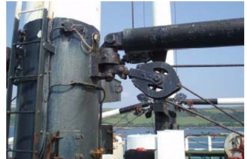
A typical derrick assembly
