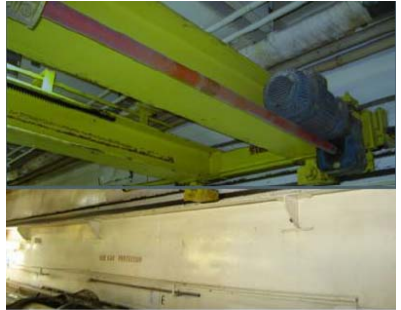
A typical engine room crane
